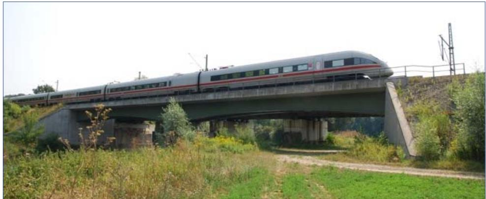
German railway company DB. Furthermore, recently developed steel trough bridges with thick floor steel slabs ( $d \geq 100$  mm) are very advantageous having, inter alia, small constructional depths and good acoustic emission characteristics.
